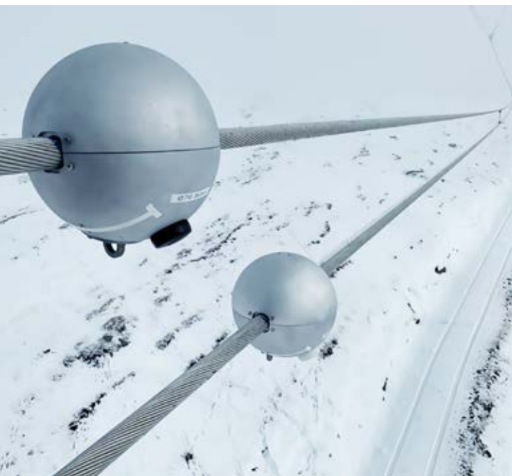
Ice monitoring sensors on overhead lines, Koralm location
