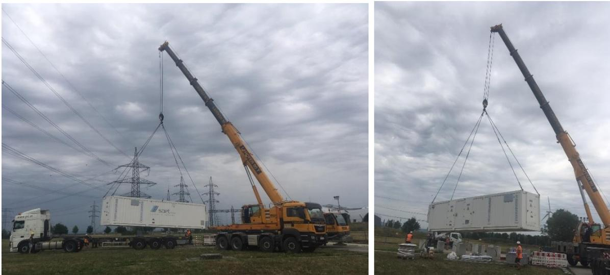
**Figure 60: Erection of the energy storage system at APG site**
